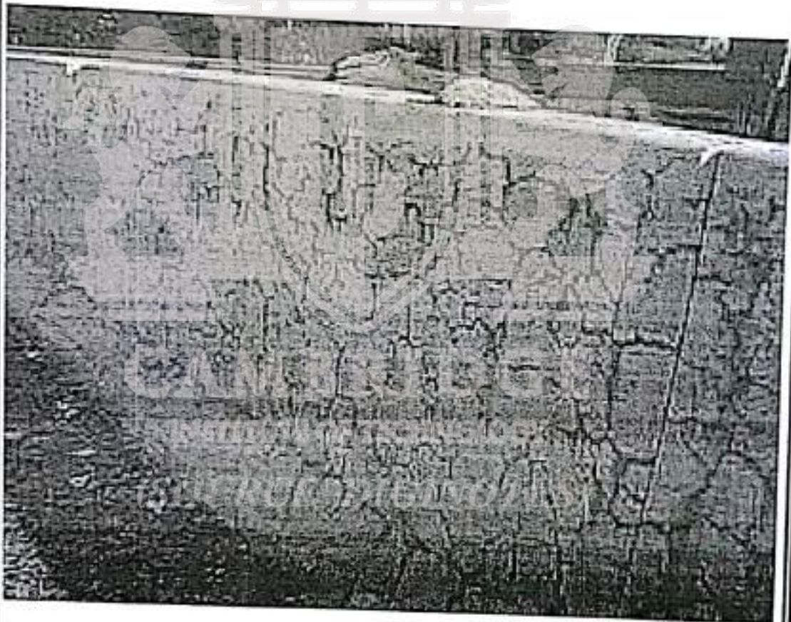
Figure: Typical effect of Alkali-Aggregate Reaction
