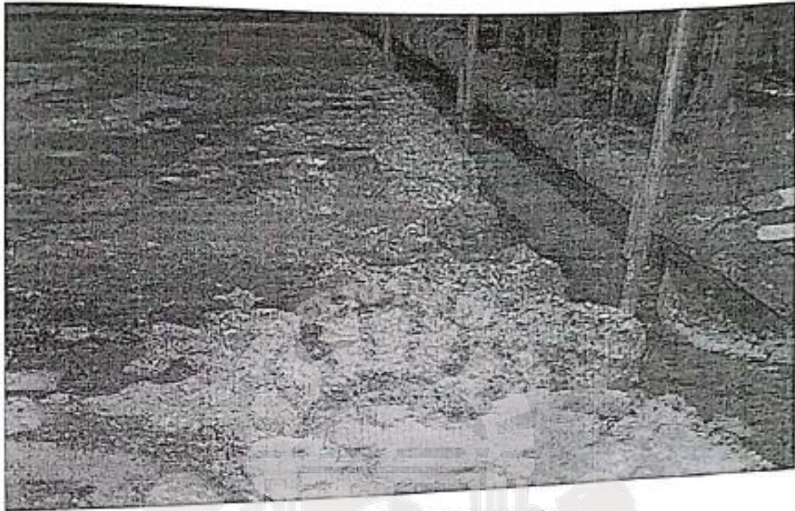
Figure: Acid attack on concrete
